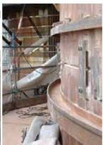
Prep completed. 'C' plates and alignment plates fitted
