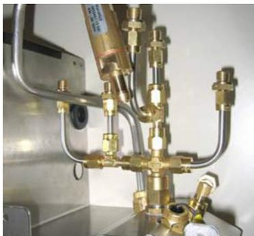
Boiler subassembly pre-fabricated by Serto, mounted and installed by customer.
